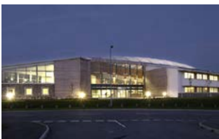
Technium Building, Pembroke Dock
